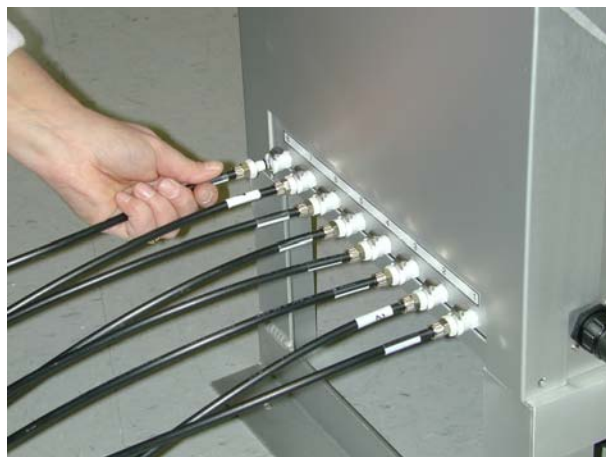
Figure 2.10 Tubing Installation (SuperSASS)
